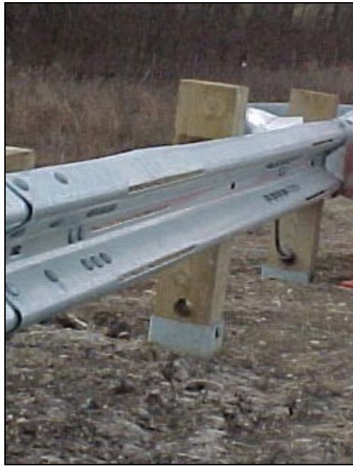
Figure 6 Slotted Rail Terminal (8)
