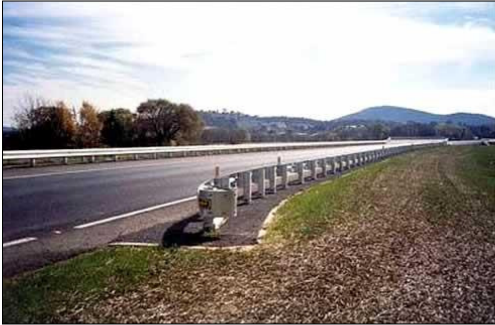
Figure 5 Modified Eccentric Loader Terminal (8)
